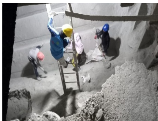
Gambar 2 Proses Cleaning Palka
